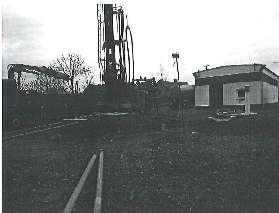
Prace remontowe na SUW Krzycko Wielkie.
